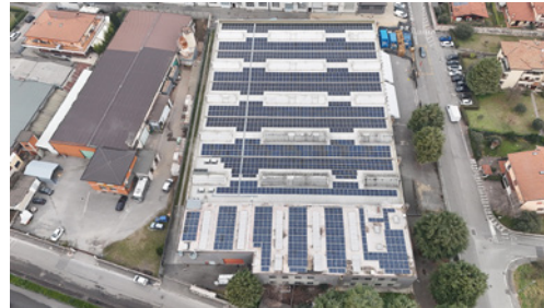
Daikin Compounding Italy S.p.A. introduced solar power generation system at its factory
