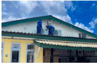
Installing an outdoor unit on a house
